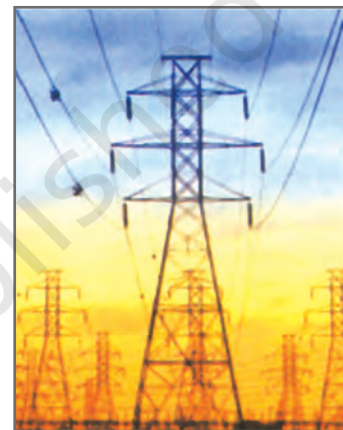
Fig. 3.7: National Power Grid to supply Electricity
